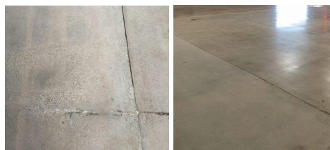
Before – Bare Concrete Surface After – Complete Hybrid/Twister Restoration
